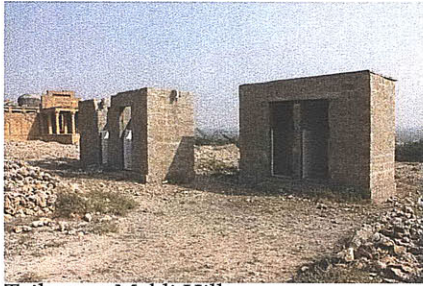
Toilets on Makli Hill
